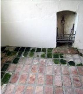
The telltale indications of excessive moisture include tide marks on walls or floors, patches of white powdery salt crystals on wall surfaces, green algae or mould growth and blistering paint or plaster. Keep an eye out for these signs as you look around your building.
